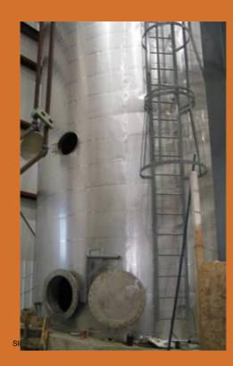
Tube & Shell Heat Exchanger
